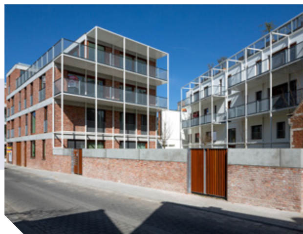
▲ CAAAP Portier 51, Malines
