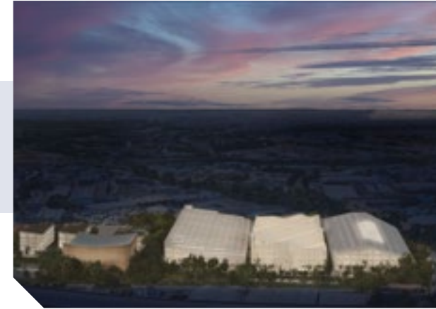
▲ Uplace SA Broeklin, Machelen TYPE DE PROJET Mixed-use ARCHITECTE ORG Urbanism & Architecture + Jaspers-Eyers Architects
